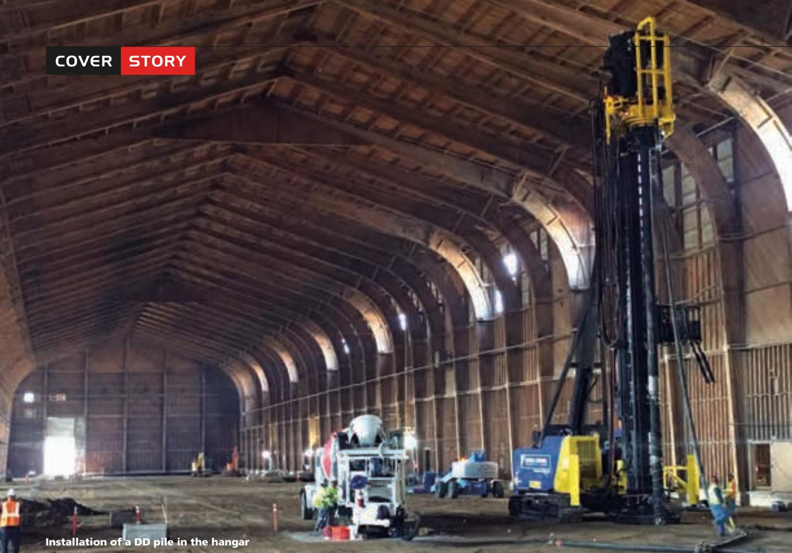
Installation of a DD pile in the hangar
