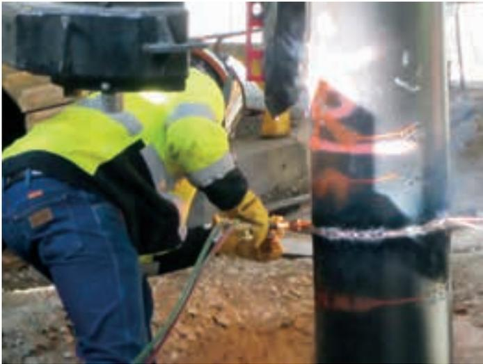
**Welding additional casing length on PC-CIDH pile**
