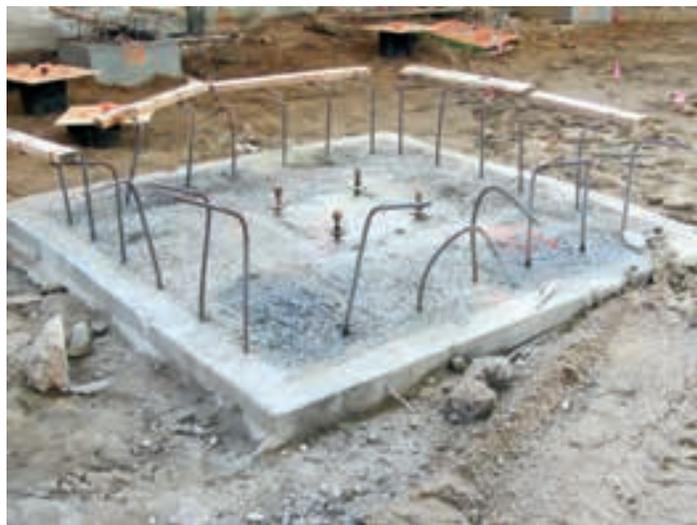
**Constructed pile cap atop PC-CIDH piles**
