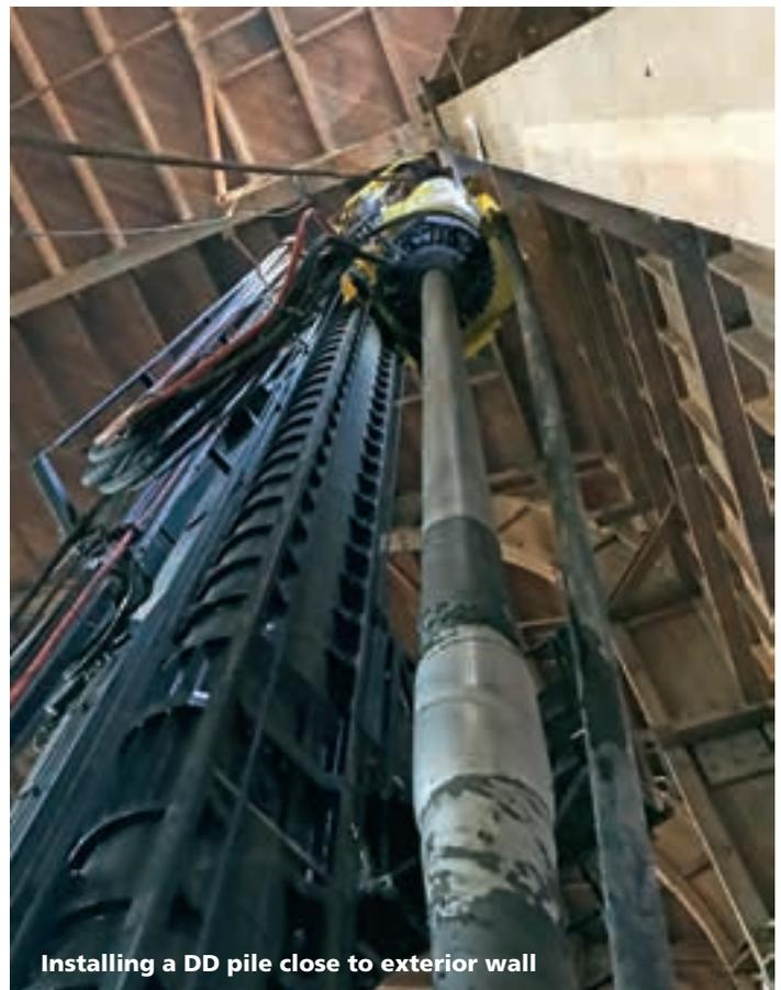
**Installing a DD pile close to exterior wall**
